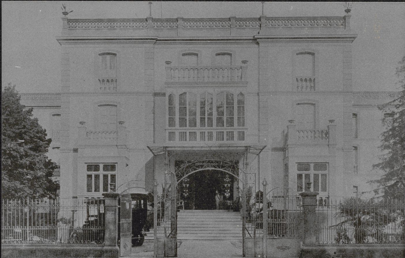
GRAND HOTEL, LOGROÑO: FACHADA PRINCIPAL
